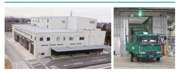
This is an intermediary processing facility that begun operations in April 2019, to process recyclable waste such as bottles and cans. These facilities are capable of processing 26 tons per day of oversize/non-combustible waste (in 5 hours), and 34 tons per day of recyclable waste (in 5 hours).
