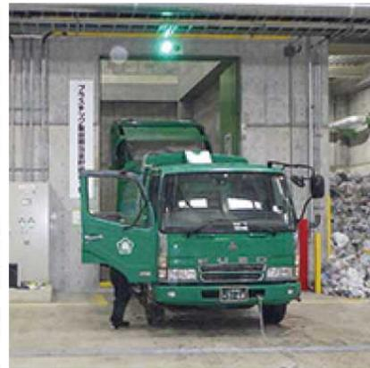
This is an intermediary processing facility that began operations in April 2019, to process recyclable waste such as bottles and cans. These facilities are capable of processing 26 tons per day of oversize/non-combustible waste (in 5 hours), and 34 tons per day of recyclable waste (in 5 hours).
